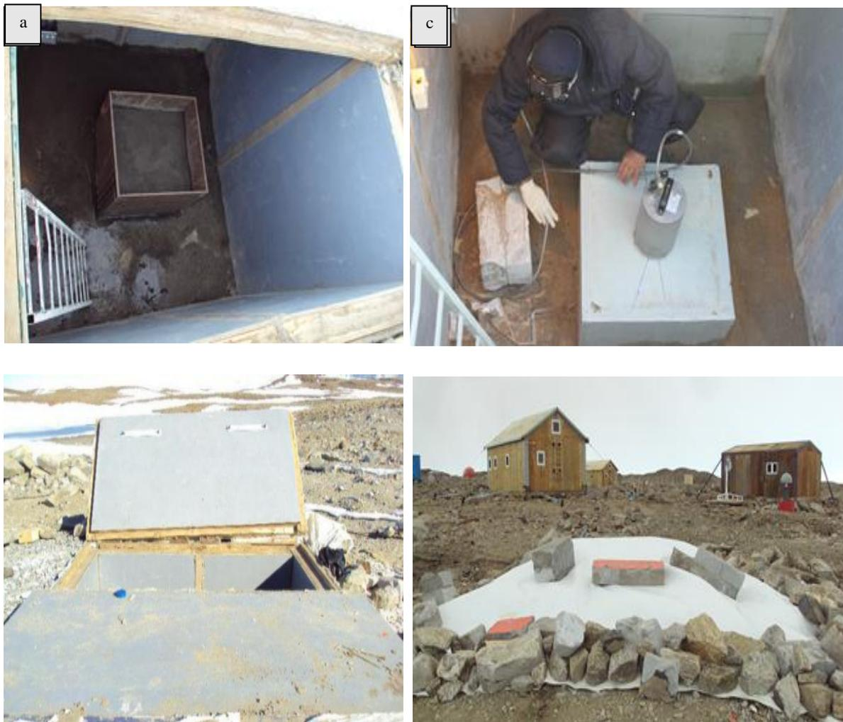
Figure 3: (a) A photo taken during vault construction for broadband seismometer (b) Top view of seismic vault platform anchored to bedrock (c) Installation of broadband seismometer (d) Photo of constructed enclosure room and seismic vault
